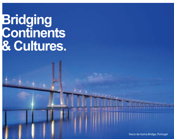
Vasco da Gama Bridge, Portugal
